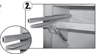
Position the drawer box in the opening so it balances on the brackets. Position the end of the slide so that it sets back from the face of the drawer box.
