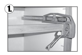
Place the brackets into the drawer box opening so that the support tabs of the brackets rest on the top of the face frame rail and under the slide as shown. Clamp the bracket to the face frame to hold it in position.
